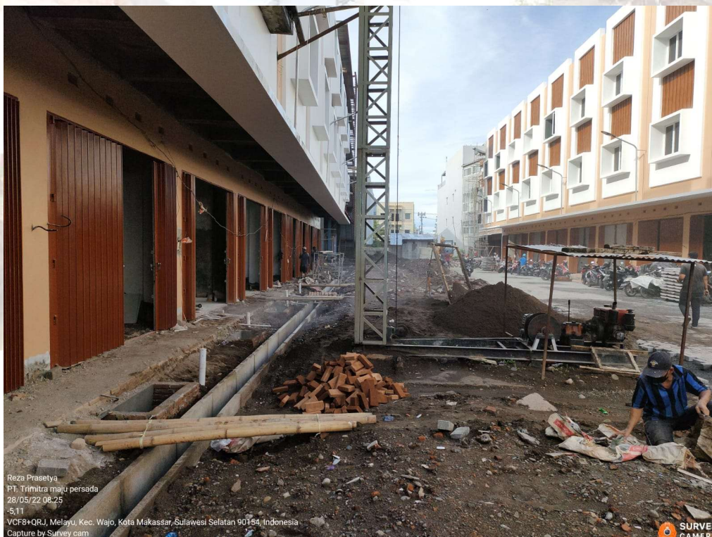
Pekerjaan Sal U-Ditch & Cover – Graha Biz Park Jl. Buru
