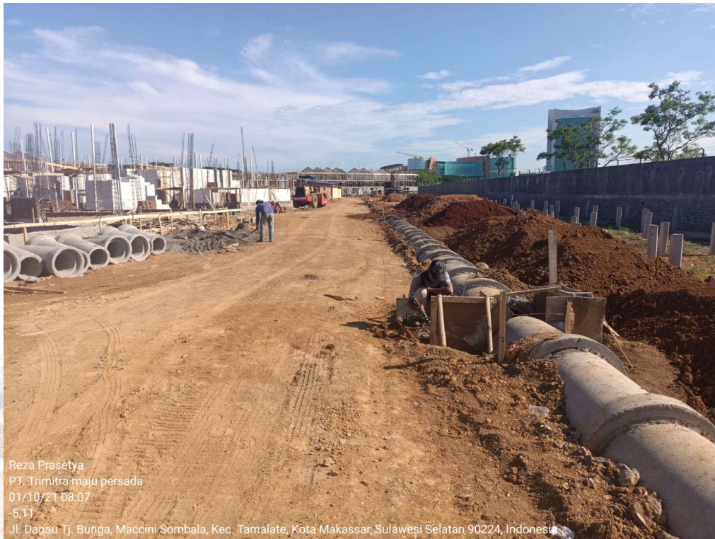
Pekerjaan Sal Rolling Hills – RKM – RCP
